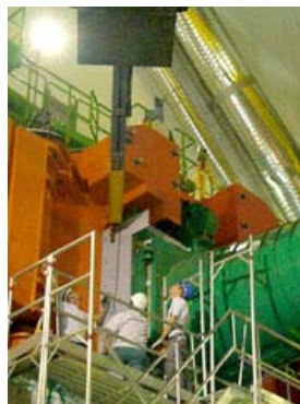
Installation of side part of FIN sealing
