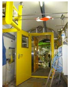
Installation of pressure resistant door in the survey gallery
