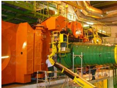
Installation of top part of the FIN sealing
