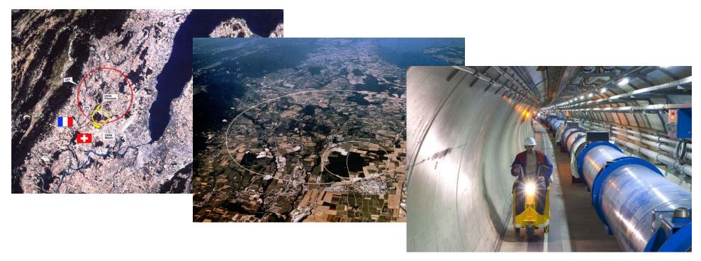
Trillions of protons will race around the 27km ring in opposite directions over 11,000 times a second, travelling at 99.99999991 per cent the speed of light.
